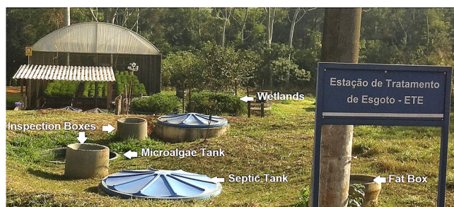
Fig. 2. Sewage Treatment Station (STS) and greenhouse.
