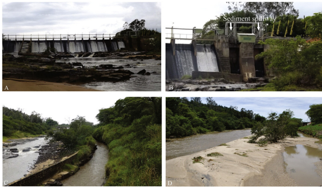
Fig. 3. (A) View of Quatiara hydroelectric, located upstream of the reaches, (B) view of the dam showing the sediment spillway, (C) channel downstream of the dam, and (D) volume of sediments mobilized by the opening of the spillway. (Available from http://www.nossalucelia.com.br/n7745.html .)
