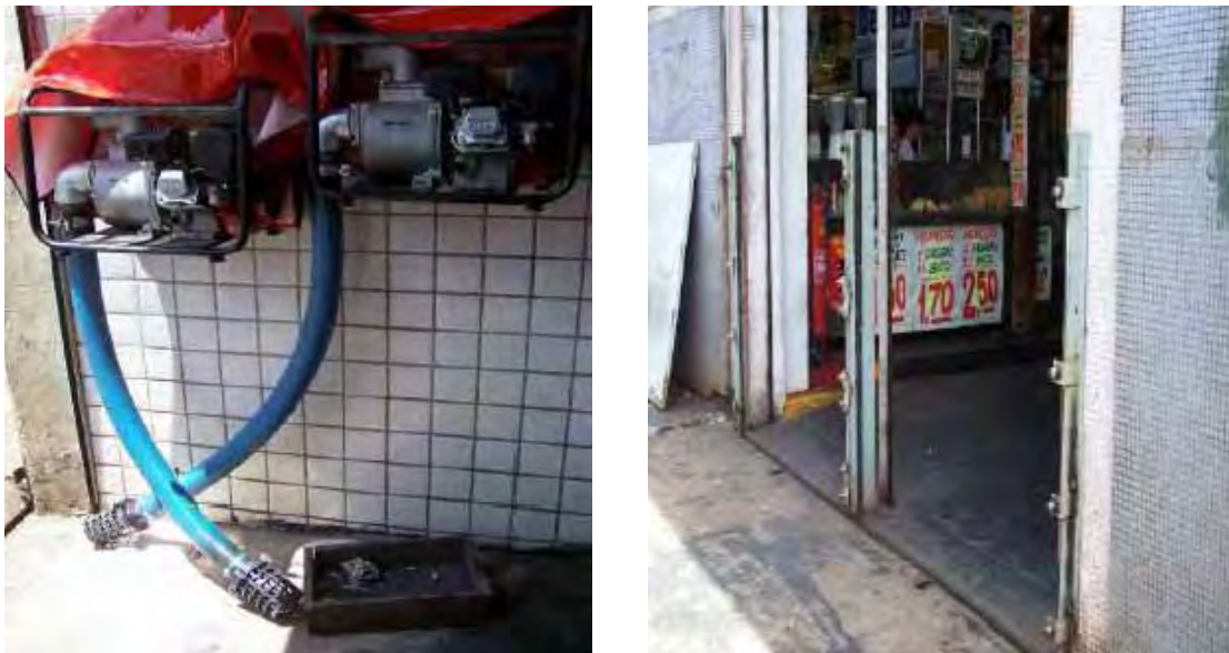
Figura 45. As bombas de água e as comportas do Mercado Municipal (Foto do autor, 10/01/2006).
