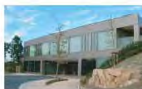
Fig. 2 The appearance of PAPI with four wall-integrated DSC panels.
