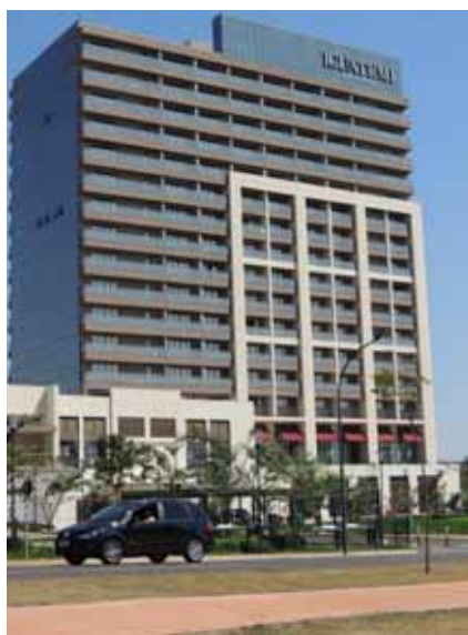
Foto 46 - Iguatemi Shopping. Torre Comercial 2014.
