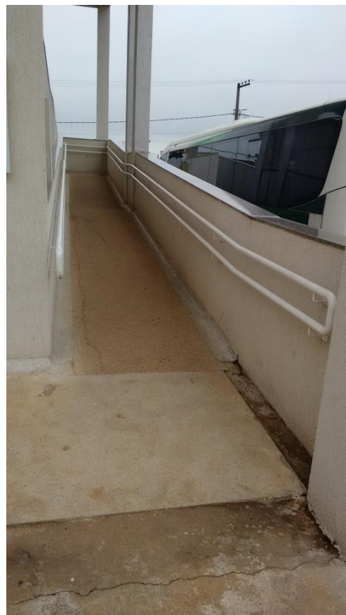
Rampa – Bloco D
