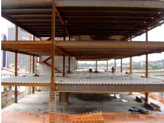
Figura 17 – Laje Steel Deck
