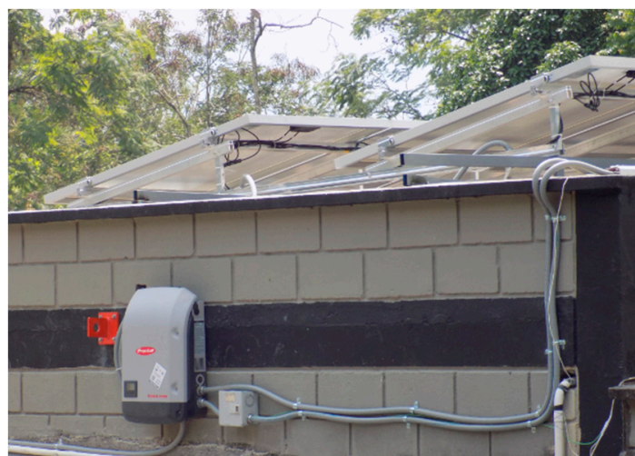
Figure 3. Photovoltaic system on-roof devices.
