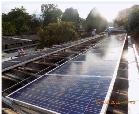
Figure 2. Photovoltaic system used.
