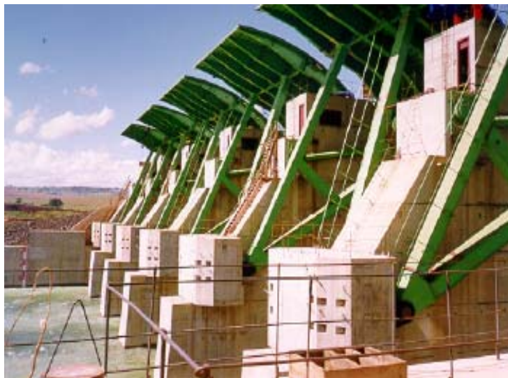
Figura 15: Comporta Segmento (ALSTOM, 2006)
