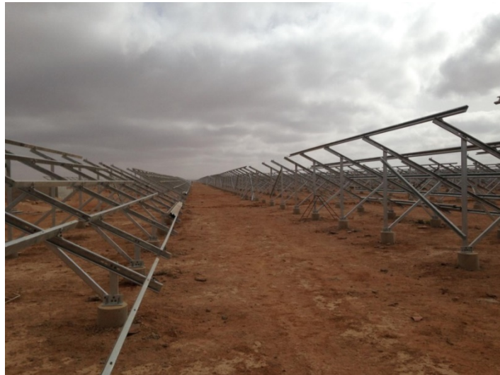
Figure 10 – A Moroccan PV power plant under construction.
