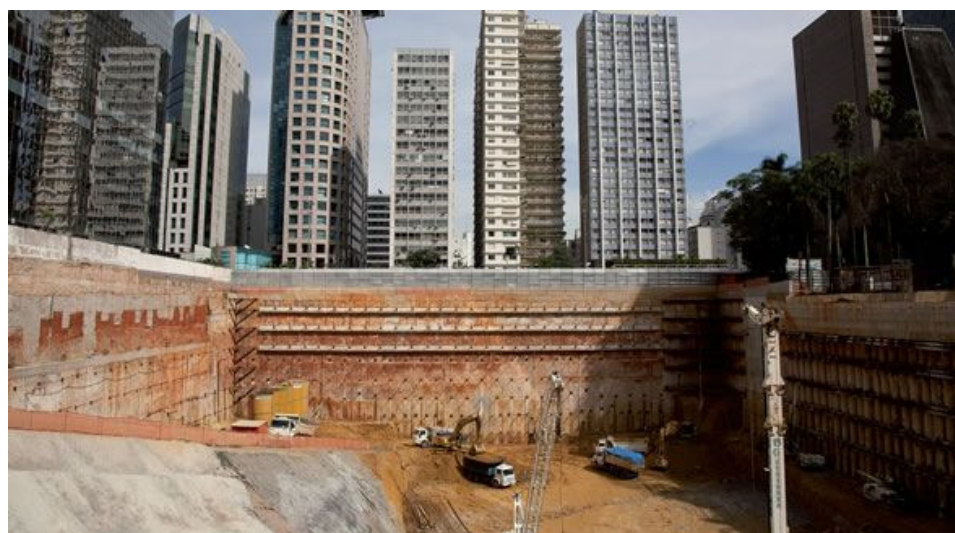
Figura 5: Parede diafragma (Techne, 2012).
