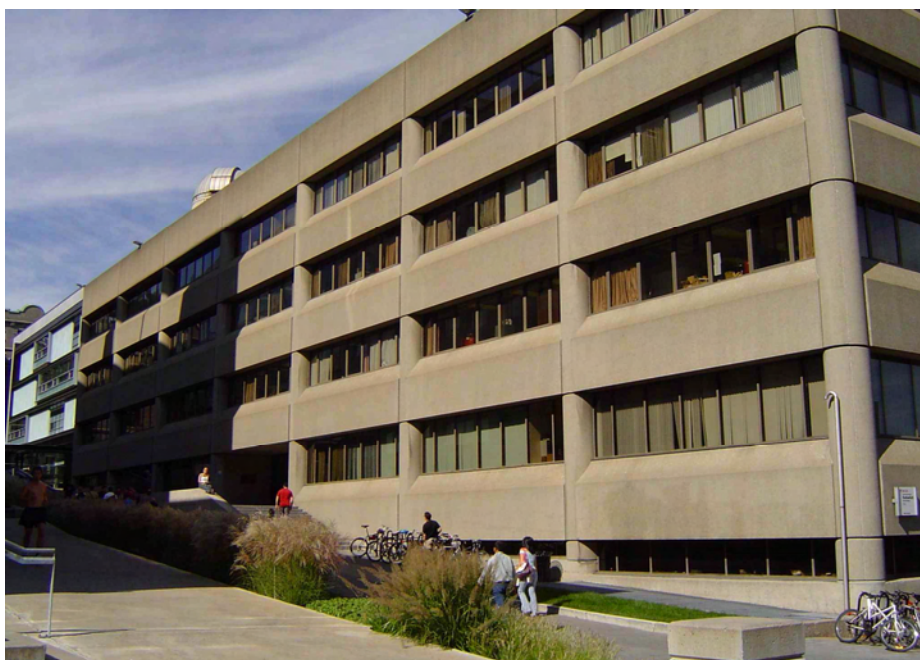
FIGURA 3.3 The Ernest Rutherford Physics Building - Universidade McGill (Foto do autor, set/2004).
