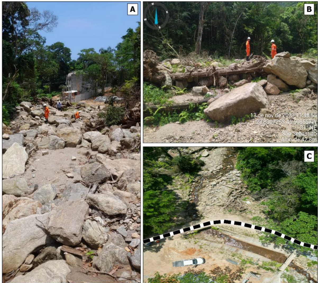
Figure 38 - Documentation of erosion caused in the main drainage by the debris flow. A) Record of metric blocks and deposits in the main drainage. B) Documentation of imbrication of large woods and metric blocks deposited in the main drainage after the passage of the debris flow. C) Aerial view of the section crossing the Petrobras pipelines where the construction managed to protect the infrastructures after the passage of the debris flow. To watch the video of the debris flow passing through this section, please access the following link: [ https://www.youtube.com/watch?v=w2EuEz2mEeo ]
