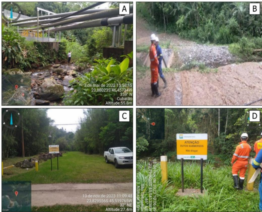
Figure 22 -Documentation of the situation of a watercourse crossing section intersected by pipelines and their respective construction patterns. A) Record of an aerial pipeline construction pattern. B) Example of a structure for the containment of potential flows in the pipeline zone. C) Crossing section segment marked with an underground pipeline. D) Section with signage indicating a submerged pipeline
