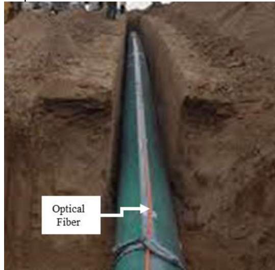
Figure 1.10 - Example of application of optical fibre.
