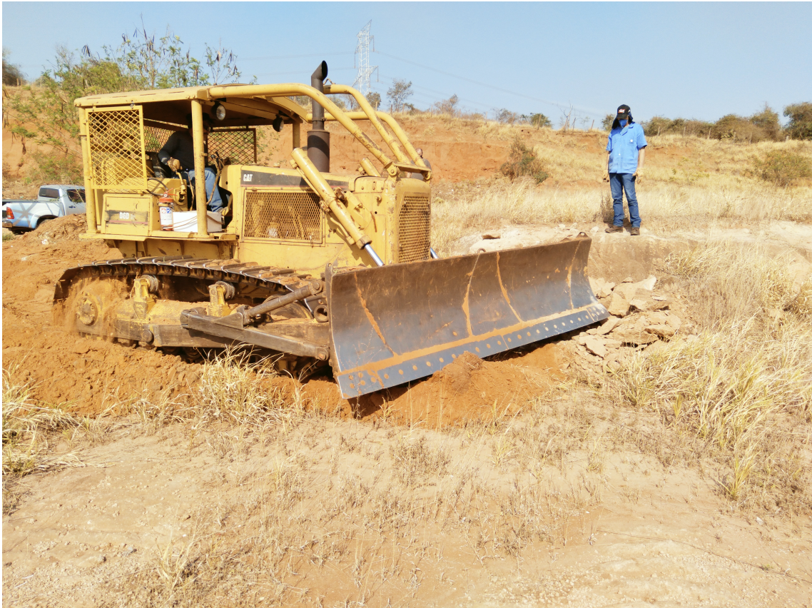
Figure 2.3: Crawler bulldozer supporting the collection of sandstone samples.
