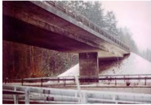
Figure 5 – View of the Z-24 Bridge.
