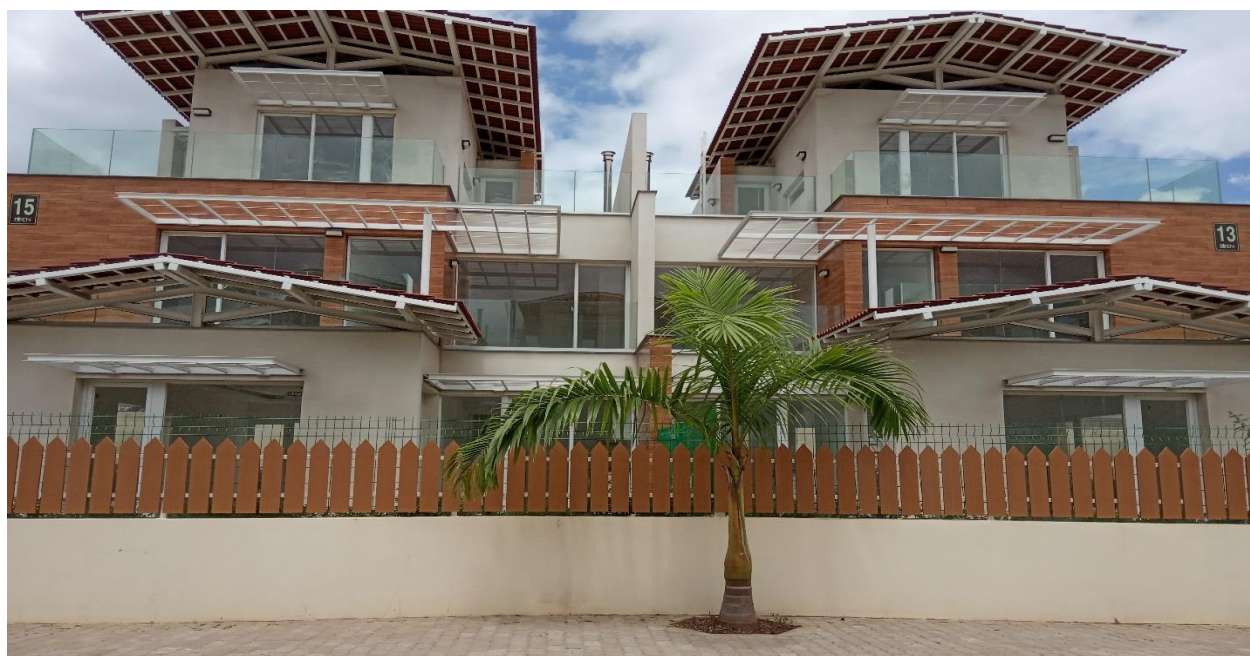
Foto 38. Vista parcial do ERF Eden Residence Gardens
