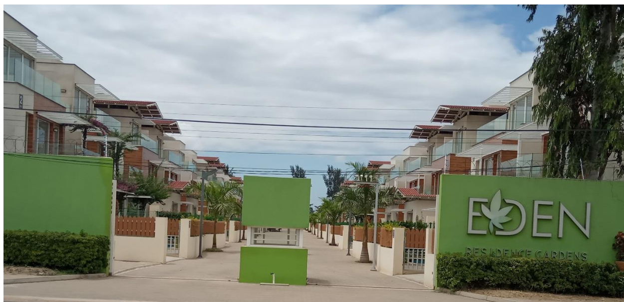
Foto 37. Vista parcial do ERF Eden Residence Gardens
