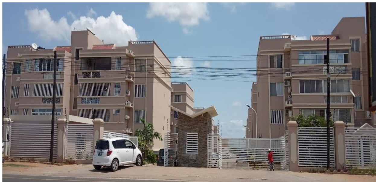
Foto 40. Entrada do ERF Kings Village Ala A
