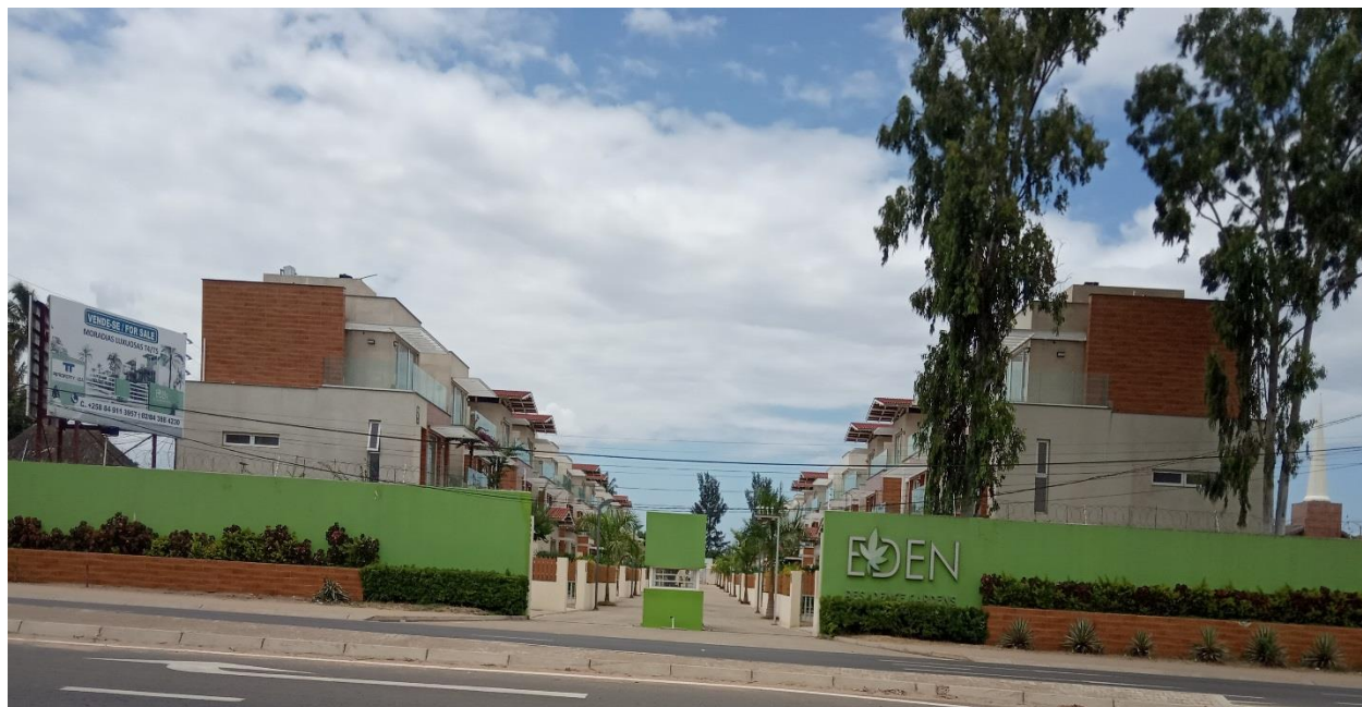
Foto 36. Vista parcial do ERF Eden Residence Gardens
