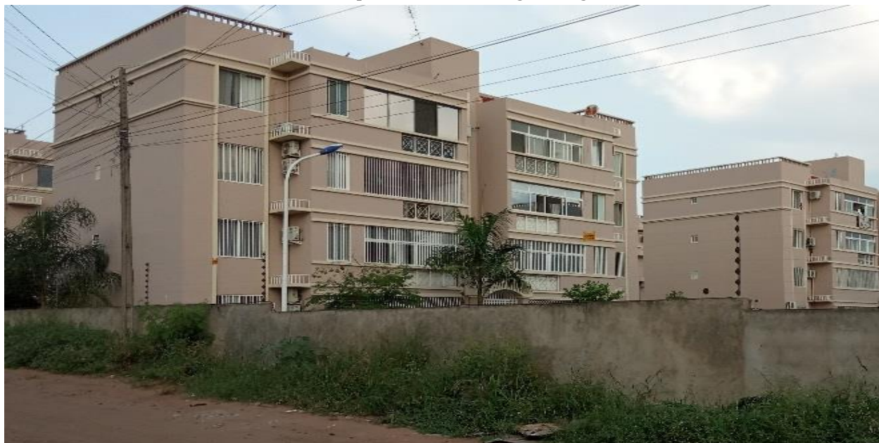
Foto 41. Vista parcial do ERF Kings Village Ala A
