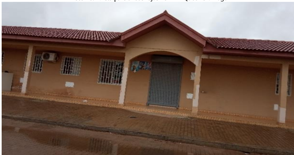
Foto 26. Vista parcial das lojas no ERF Queen's Village
