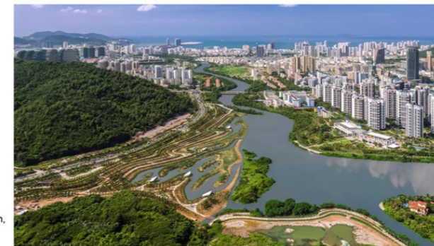
The process of construction, April 2017
