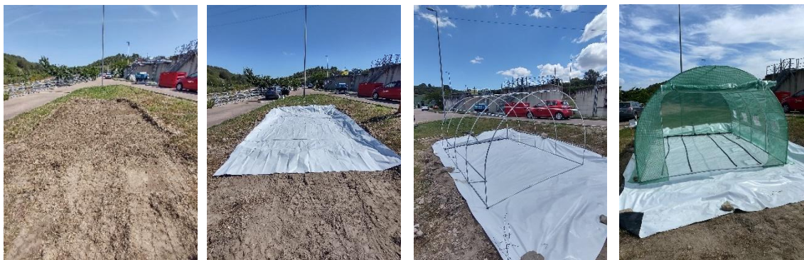
Fig. 32, 33, 34 and 35. Leveling the ground; installation of the white waterproof tarpaulin; assembly of the greenhouse structure; and greenhouse finished and ready for the start of the experiment.
