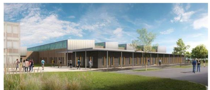
Figure 5 - Construction ateliers de formation lycée Henri Sainte-Claire Deville Issoire (63)
