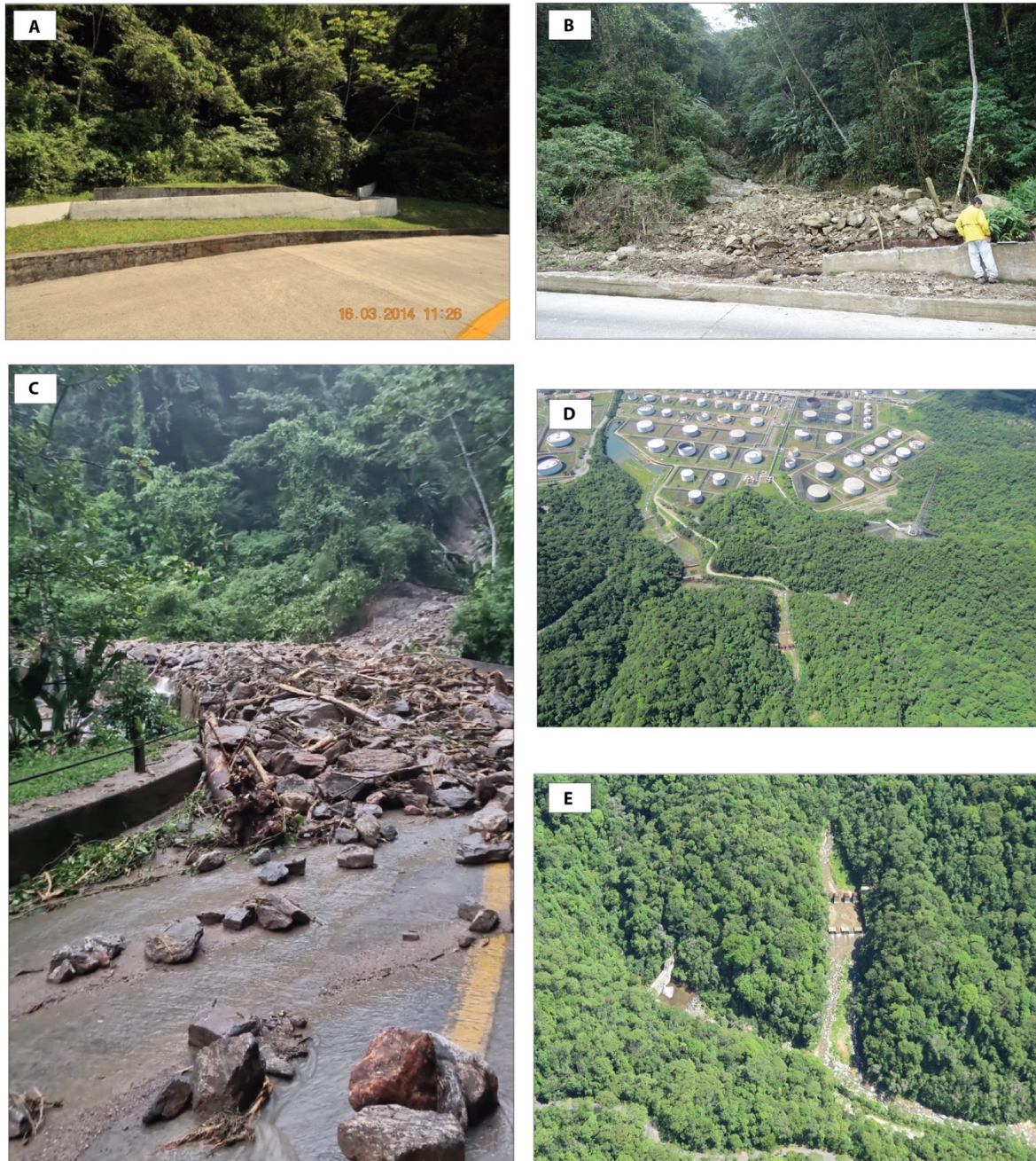
Figure 3-22. Recent debris flow in Cubatão and retention structures installed in Catchment 17. A) The tributary of Catchment 17 before the March 2022 event. Photo from 2014. B) The tributary after the debris-flow event, showing the intense erosion of the channel and vegetation. The measured post-event channel width is of 7 m. Photo from July 2022. C) Photo of the debris-flow event on the day after its occurrence (March 30, 2022). Photo from Maicon, one of the monitors of the “Caminhos do Mar” Park. D) Retention structures installed in the downstream portion of catchment 17, to protect the oil refinery from debris-flow events. Photo from Marcelo Gramani. E) Detail of two Sabo dams located in catchment 17. Photo from Marcelo Gramani.
