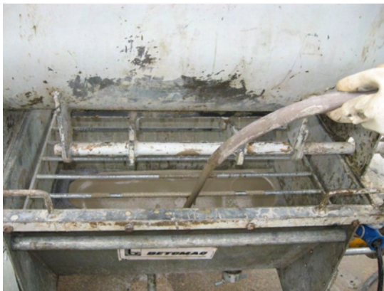
(c) Graute na betoneira
