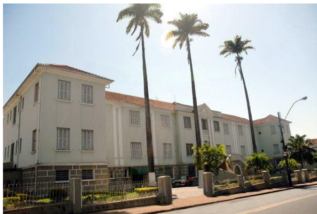
Figura 11 – Hospital Unimed II
