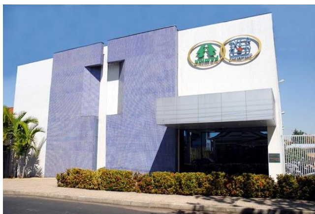
Figura 10 – Hospital Unimed I
