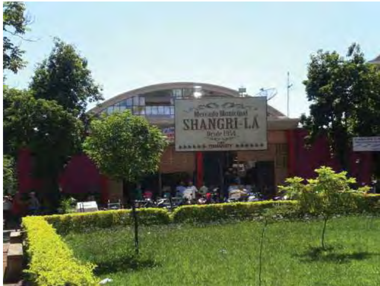
Figura 11 – Fachada Principal do Mercado Shangri Lá [Fonte: http://v8.cache4.c.bigcache.googleapis.com/static.panoramio.com/photos/original/10920895.jpg?redirect_counter=1 .]
