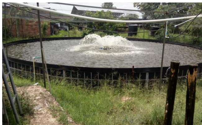
Fig. 1. Tank equipped with radial-type splash aerator
