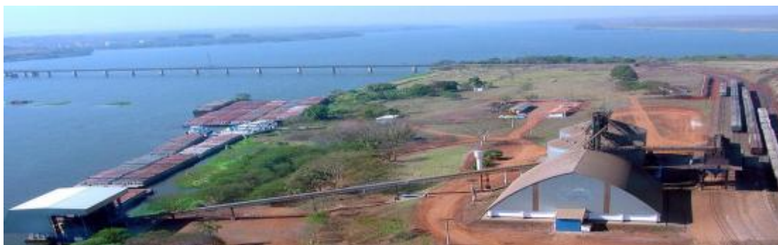
Figura 12 – Terminal multimodal de Pederneiras-SP
